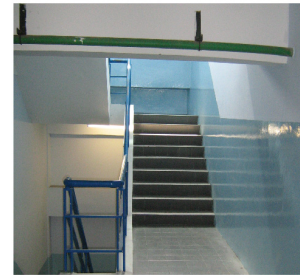
Dinding Area Tangga Darurat
